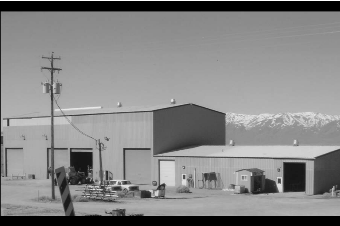
X-Cal's Secure Core Storage Facility at Sleeper.
